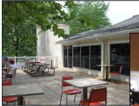
More views of the Edgemere Lodge Renovations
